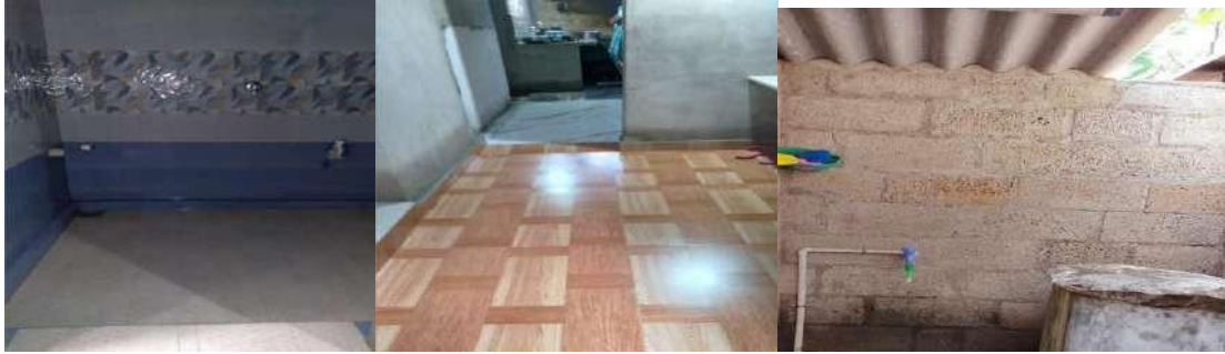
Renovations under progress
